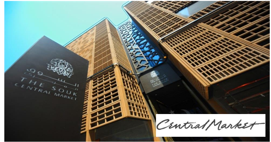
CENTRAL MARKET - Abu Dhabi Supply of Mechanical Lock Cases
