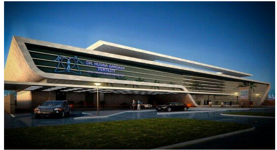
GARGASH HOSPITAL- Dubai Supply of Complete Ironmongery & Doors
