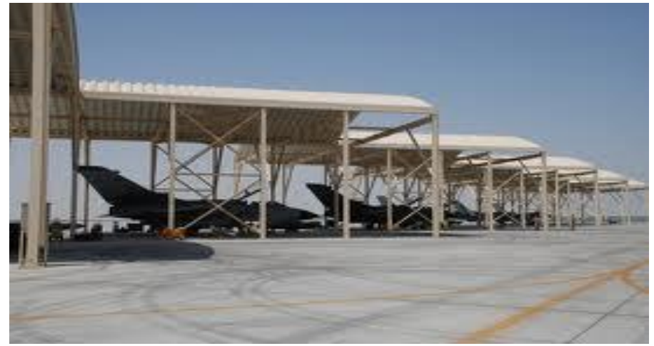
AIR BASE- Abu Dhabi Supply of Complete Ironmongery
